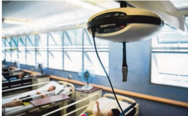
The Red Cross Home for the Disabled is using a \$130,000 manually operated ceiling track system, where the hoist can be navigated sideways.
